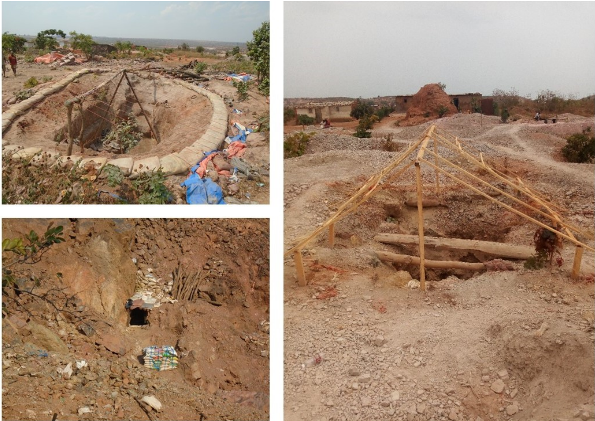
Figure 21. The pictures show rudimentary, partly insufficiently implemented safety measures at the entrances of galleries and shafts. It can be seen that in the rainy season, tarpaulins usually cover the shafts to prevent the ingress of rainwater and destabilisation of the shaft entrance.
