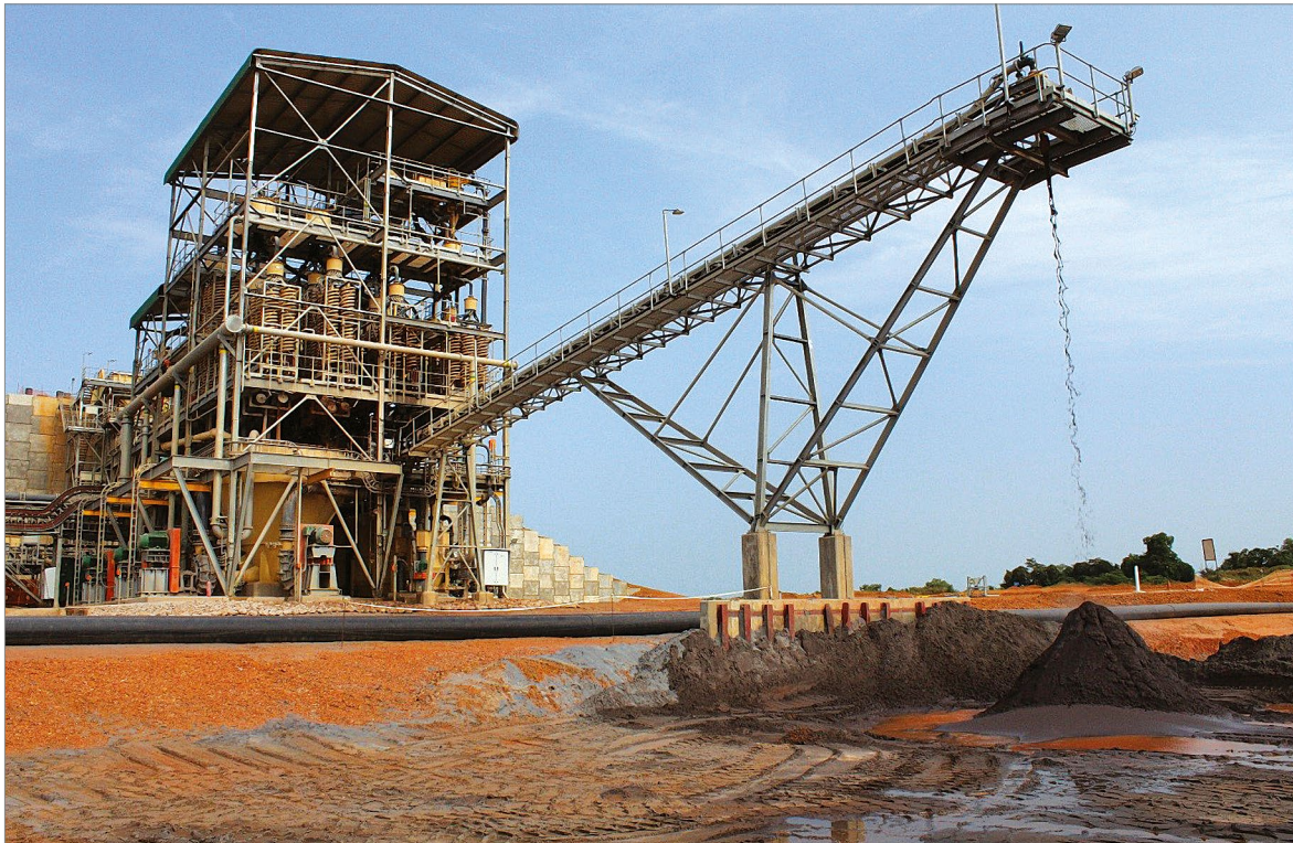
Figure 31: Photo of the Gangama processing plant in Sierra Leone. Source: Iluka Resources Ltd.
